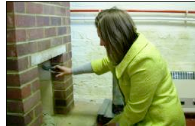
Above: Katie Elizabeth Hewer and Sandra Jones carry out safety tests for NVQ Level 3 in Domestic Gas Installation and Maintenance
